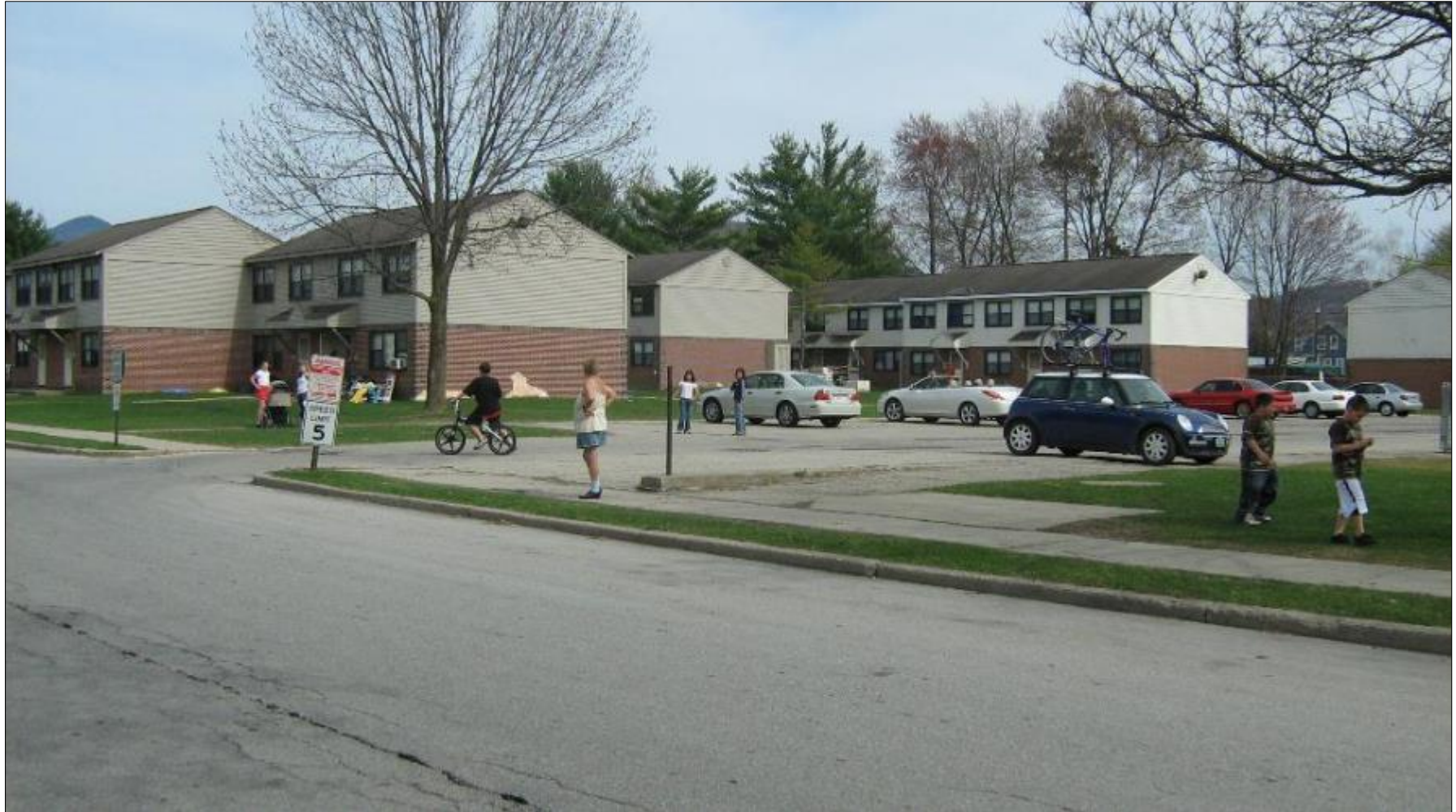
Forest Park (Rutland) - before construction
