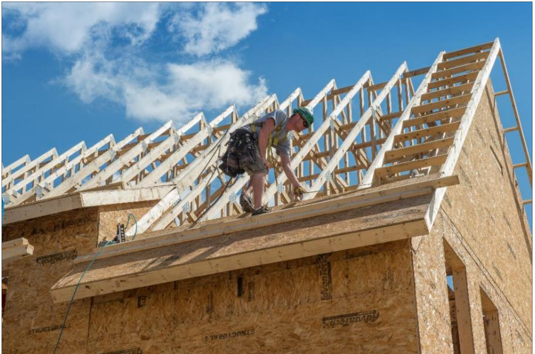
Hickory Street (Rutland) - Construction photos
