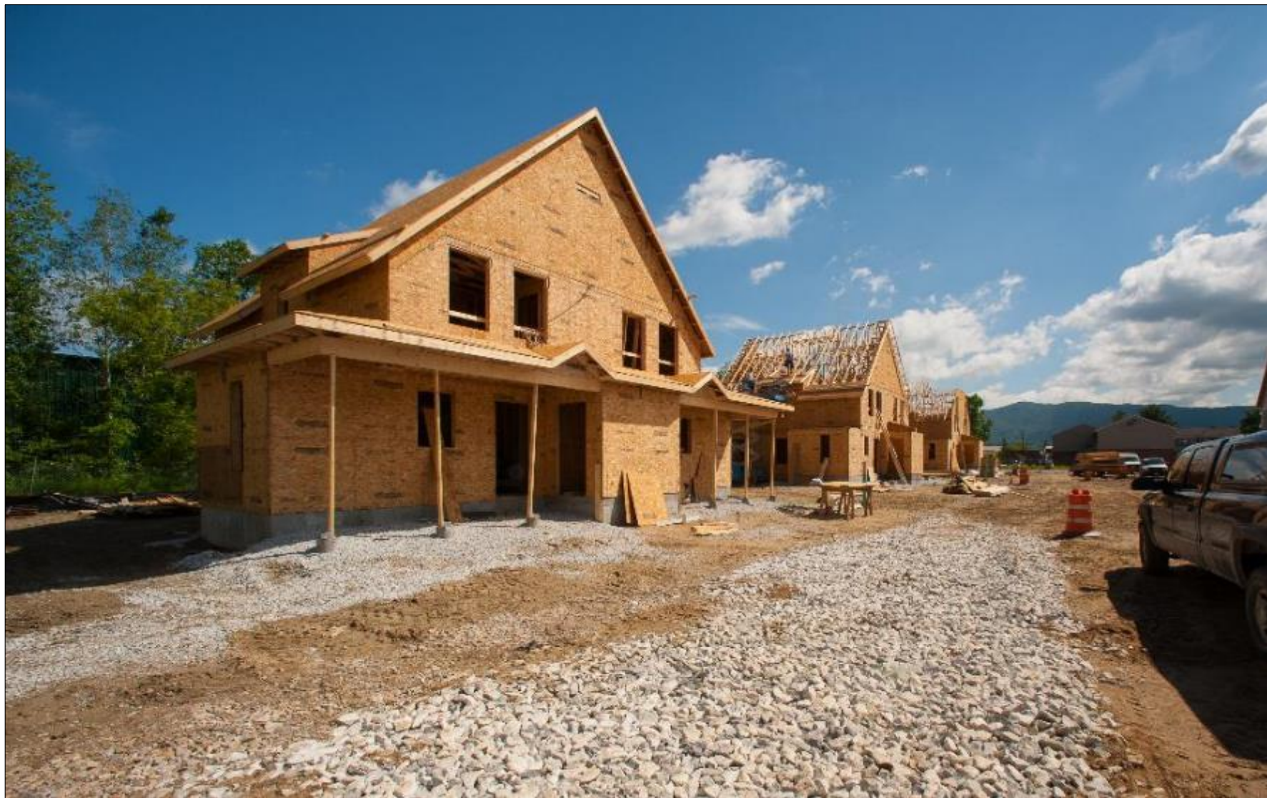
Hickory Street (Rutland) - Construction photos
