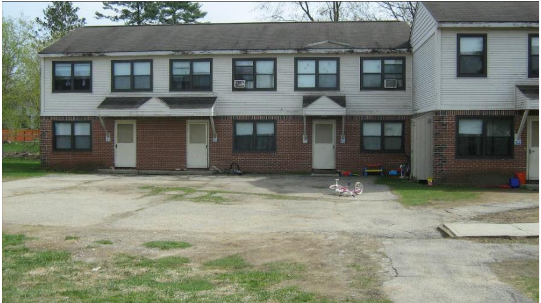
Forest Park (Rutland) - before construction
